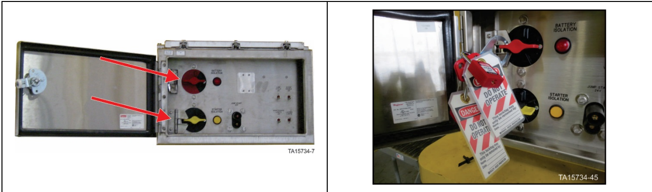
Isolation and Control switches assembly – Battery isolation switch in OFF position with locks in place
