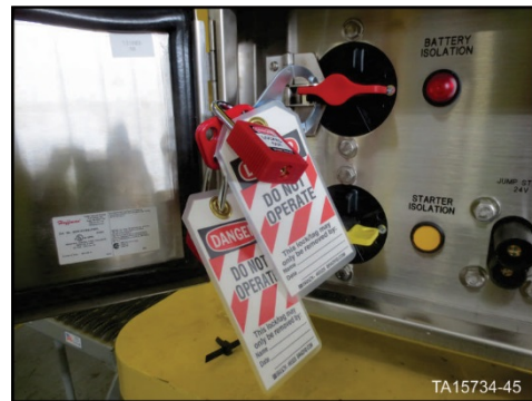
Battery Isolation Box – Battery isolation switch in OFF position with locks in place
